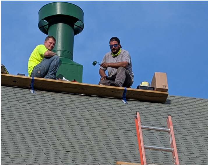
Austin Dionne and Nicholas Lasorsa painting the roof vent
