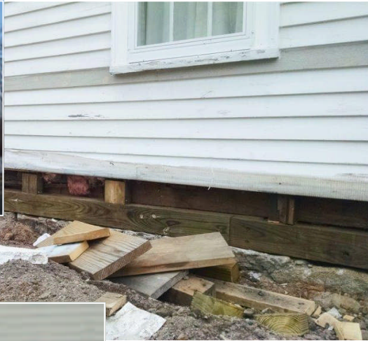
Stabilizing the foundation sill
