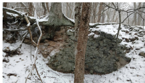
Tree roots growing into the walls on a kiln.
